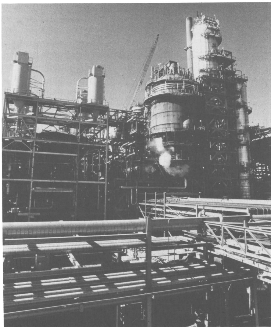
Figure 19. Commercial RCC Process Unit Reactor and Regenerator
